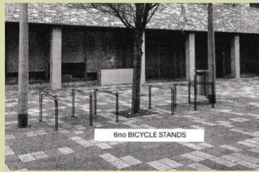
New cycle racks in the pedestrianised area of Tercott Road
