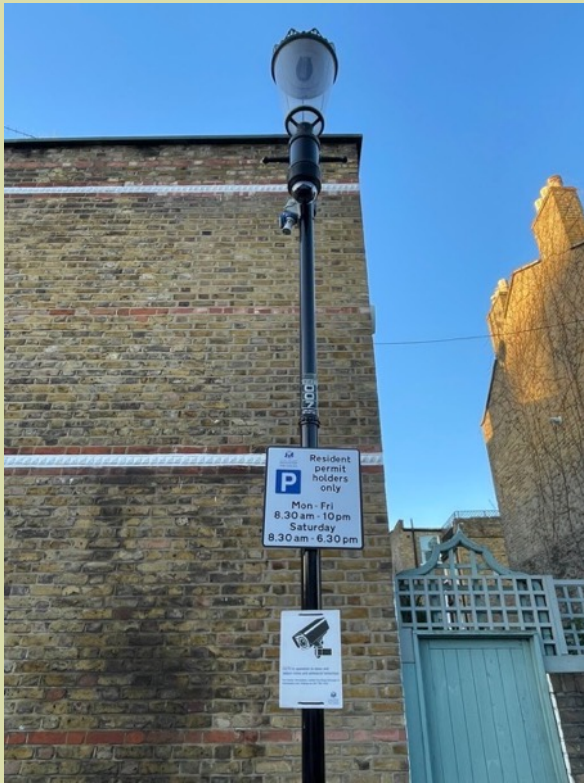
First CCTV camera installed in Tadema Road
